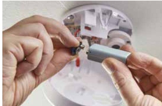
Smoke and carbon monoxide detectors
